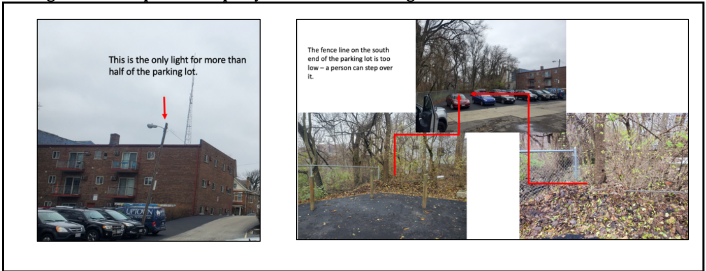
Figure 5: Examples of Property Assessment Findings at 2404 Ohio
