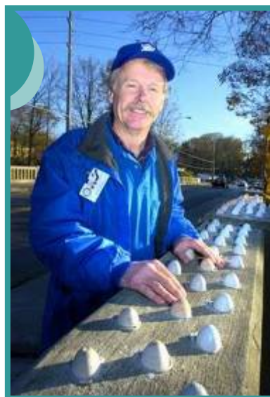
“King of the Bumps” Ben Pipkin showcases his innovative concrete eggs designed to deter loitering on the Kennedy Avenue Bridge.
