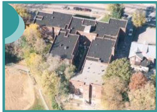
The courtyard in the middle of this 95-unit complex, a high-traffic area hidden from the street, used to be a haven for illegal activity. Citizens and police formed a strong partnership to drive out drug dealers: community members allowed CPD on property to take pictures of drug activity, the fire department turned over floor plans, and a printing company enhanced the diagrams.
