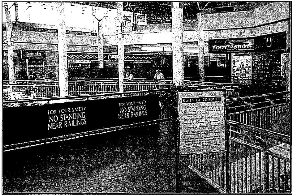
Upper Level Pedestrian Bridges with signage
