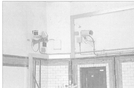
Figure 1. Conspicuous CCTV cameras cover as much of the station public areas as possible.
